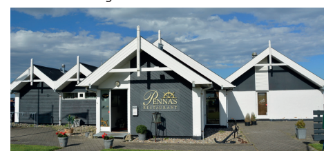
Restaurant - privat toilet
